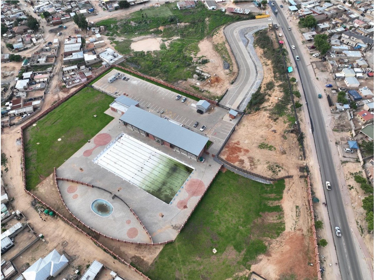
Ivory Park Swimming Pool, Off the Freedom Drive (25°59'54.40"S 28°11'44.23"E), Ivory Park Ward 111
