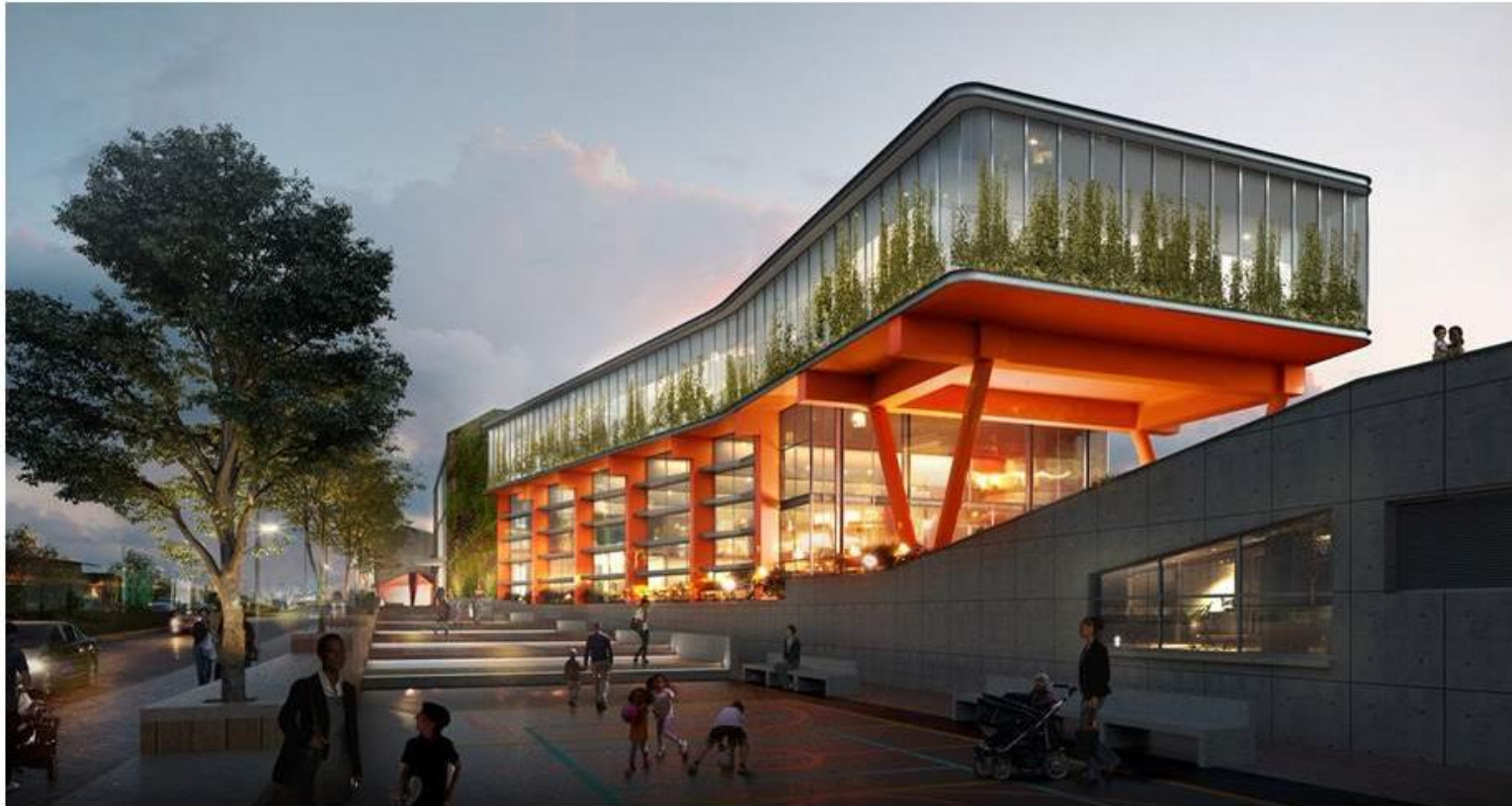
The Westbury Transformation Development Centre (WTDC). Winner in Architectural Design: Mixed Use Architecture at the 2019 Architecture MasterPrize (AMP) awards. Implemented by the Johannesburg Development Agency (JDA) on behalf of the City of Johannesburg
